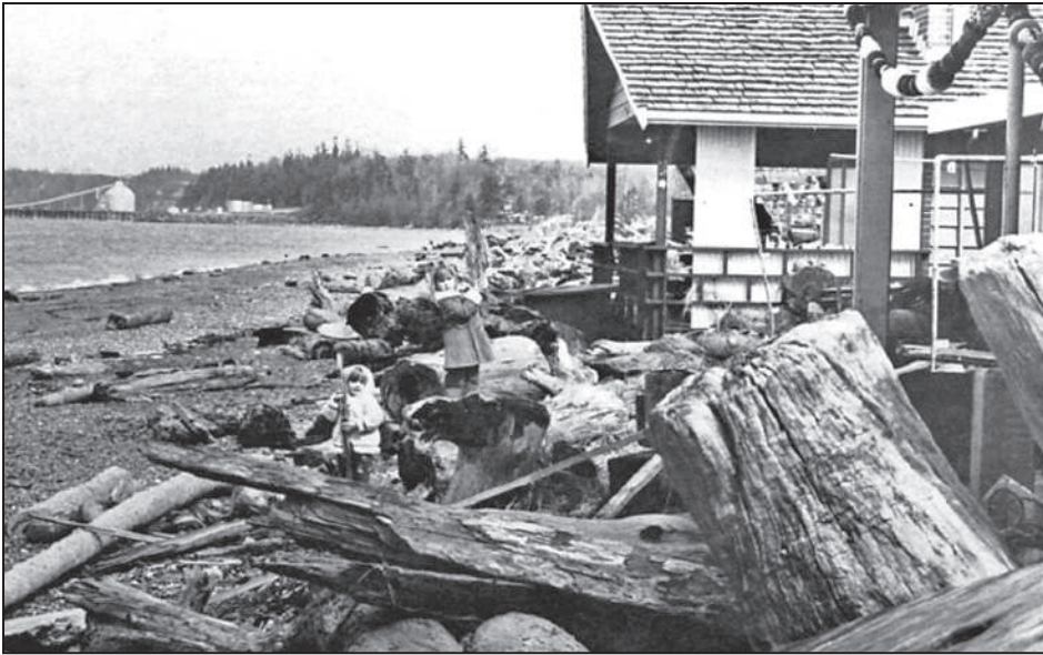
Figure 3-30. Drift logs driven into coastal houses at Sandy Point, WA, during a March 1975 storm
