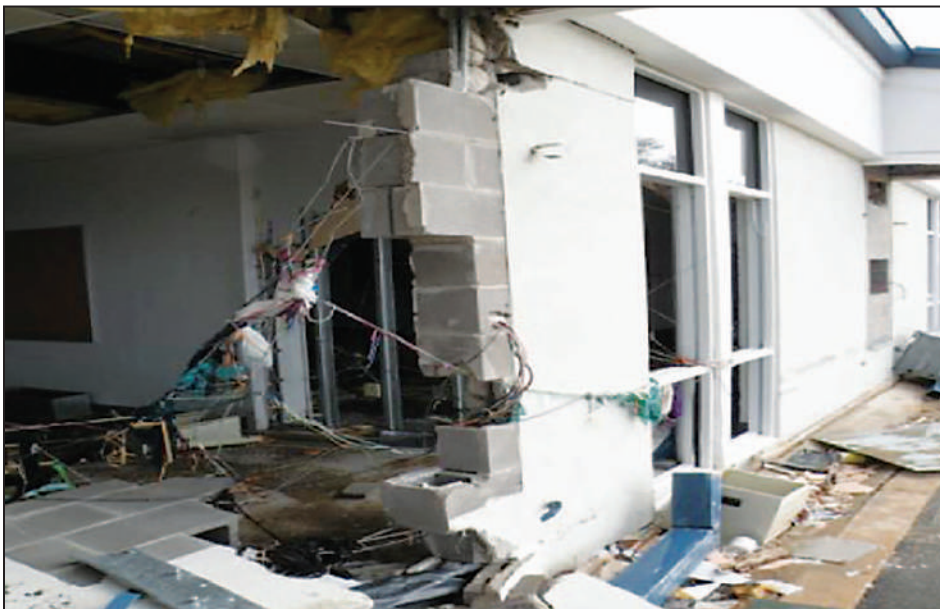
Figure 2-10. School located approximately 1.3 miles from the Gulf shoreline damaged by storm surge and small waves, Hurricane Ike (Cameron Parish, LA, 2008)
